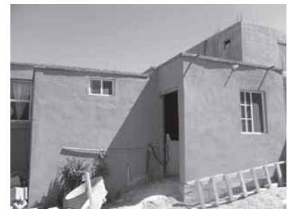
An example of a completed family dwelling.
